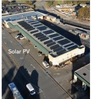
Transperth's first electric bus begins service on Joondalup CAT route powered by Tesvolt energy storage technology. The flagship project is designed using a high voltage EV fast charging station, 100 kW solar power array and Tesvolt 307kWh High Voltage Battery Storage System. The modular Tesvolt battery system is capable to store the surplus Solar PV energy generated during the day and can be discharged by the Electric CAT buses when returned to the depot.
