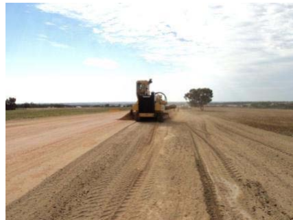
Vemeer trenching machine in operation
