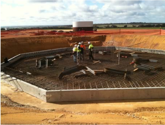
Excavation of the foundation
