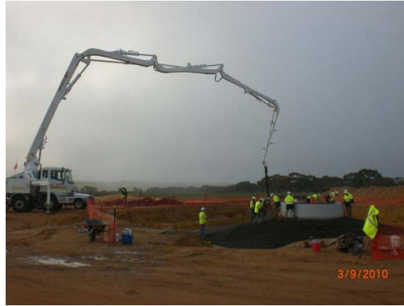
Pouring the concrete
