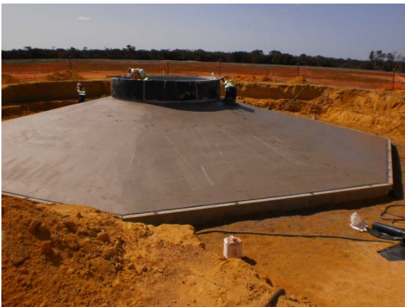
Completed foundation (close-up)
