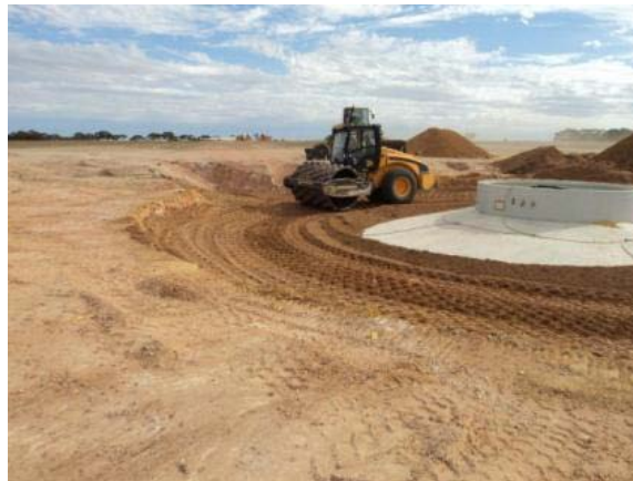
Sheepfoot roller compacting around the foundation
