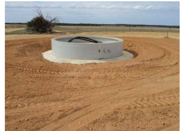
Foundation compacted
